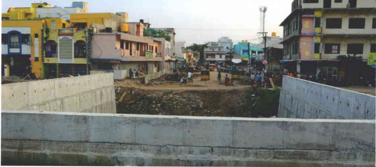
VIEW OF PADI SIDE APPROACH (WORK TO BE STARTED)
